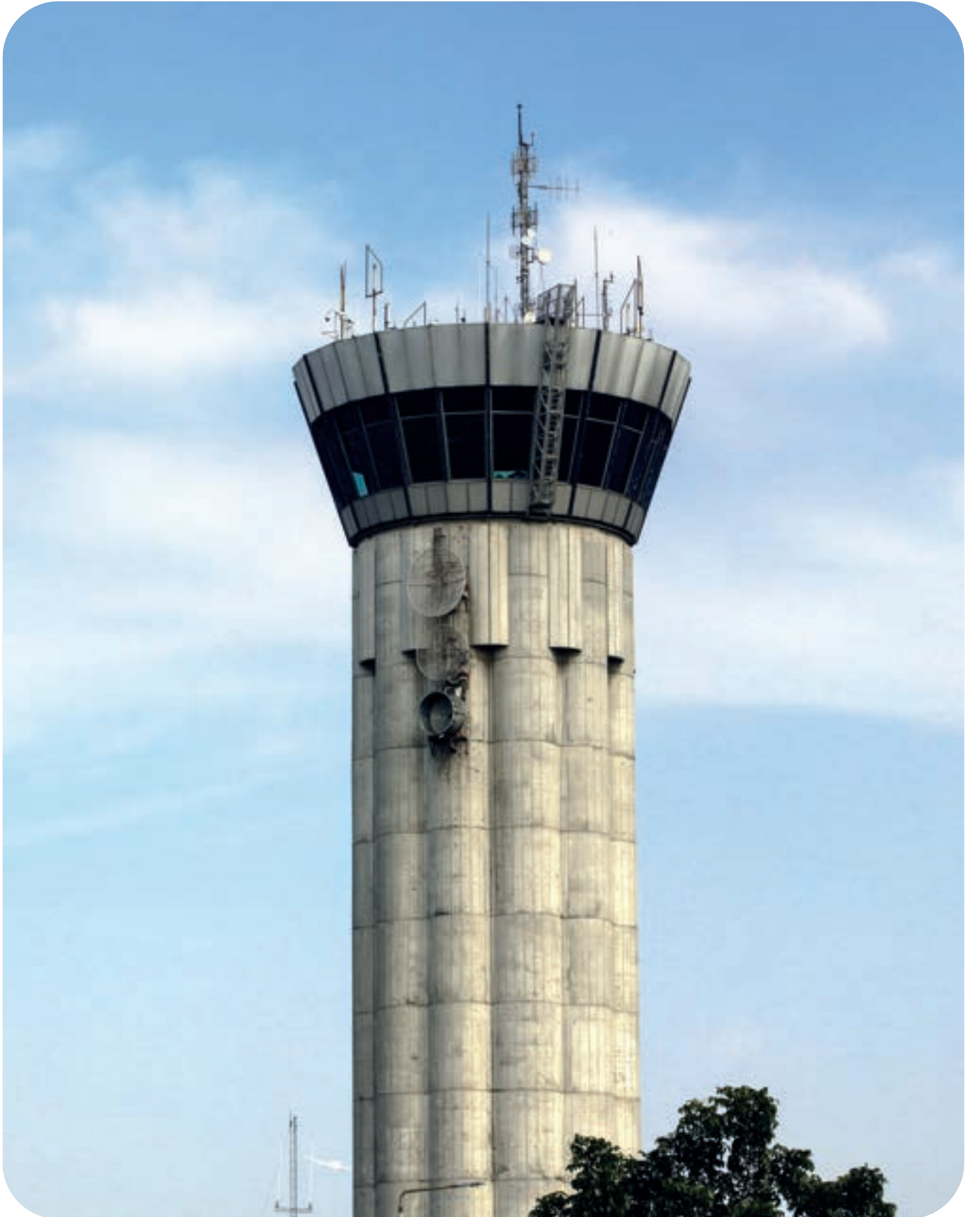
▶ Tower AirNav Indonesia Kantor Cabang JATSC. The AirNav Indonesia tower at the JATSC Branch Office.
