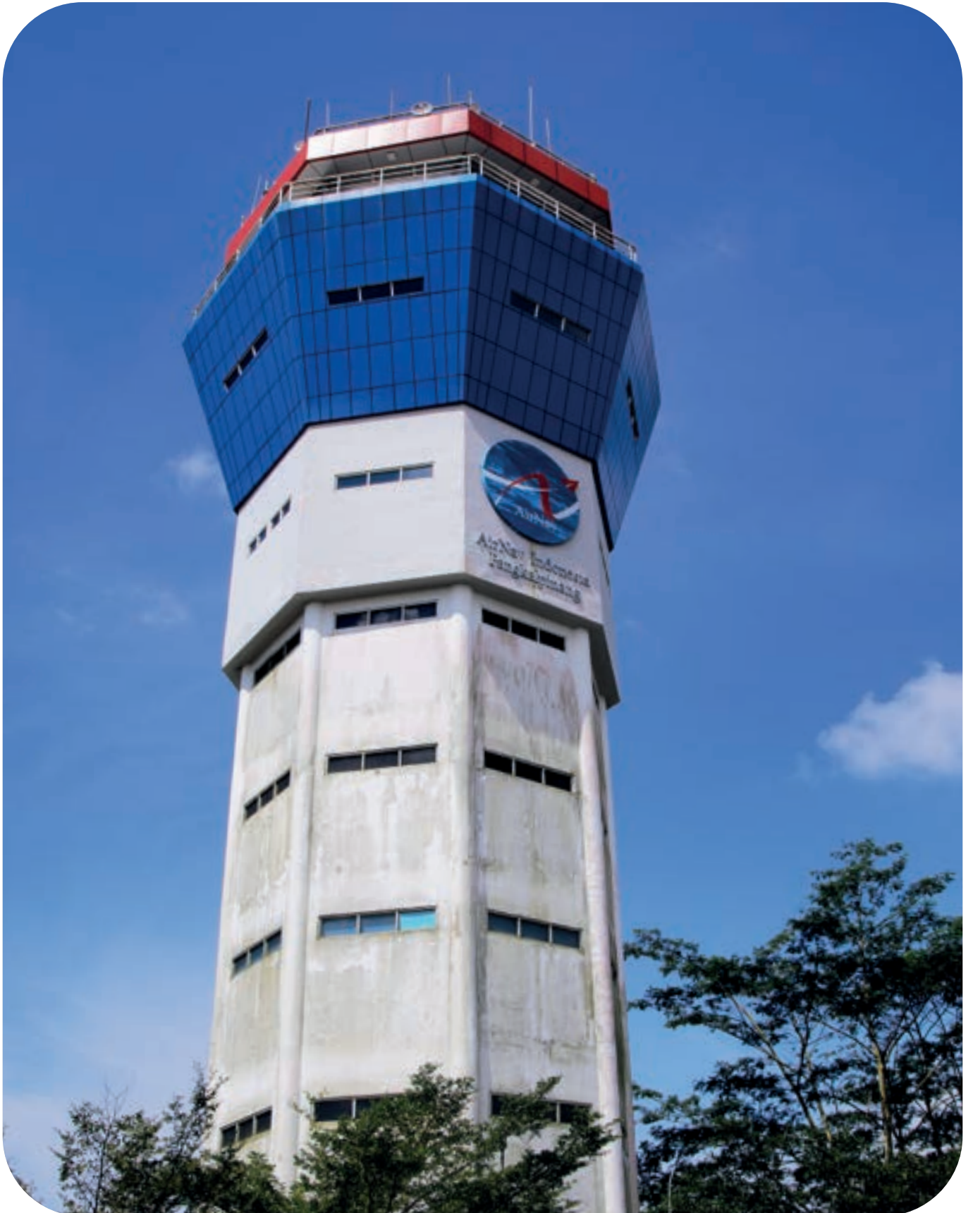
► Tower Airnav Kantor Cabang Pembantu Pangkal Pinang. The AirNav Indonesia tower at the Pangkal Pinang Sub-Branch Office.
