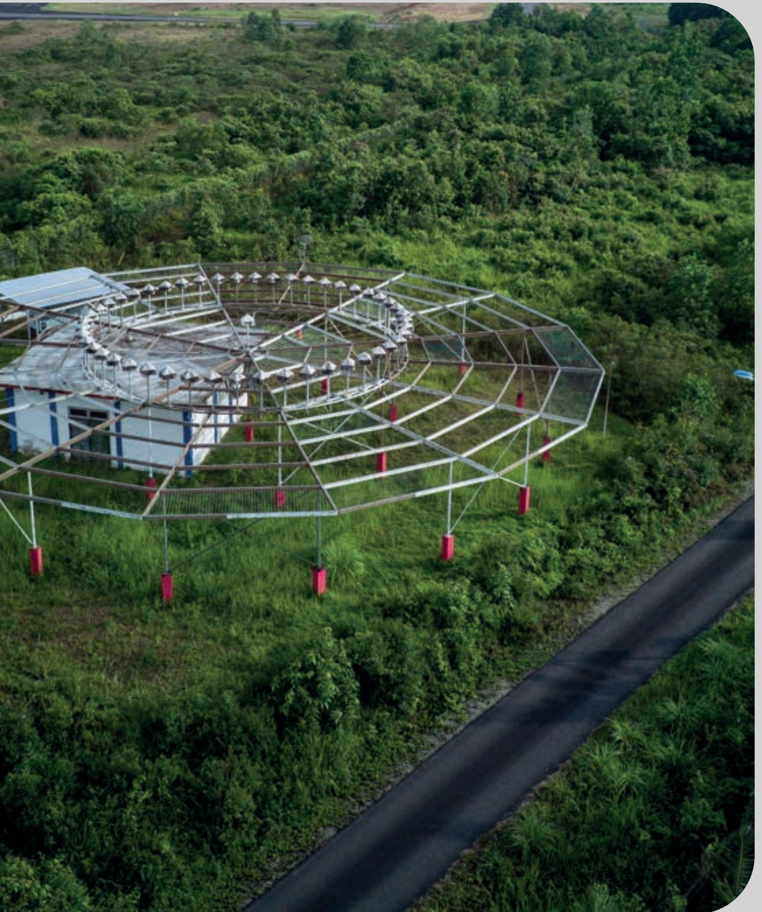
Perangkat navigasi DVOR (Doppler VHF Omnidirectional Range) yang berfungsi membantu pilot menentukan arah dan posisi pesawat terbang di Kantor Cabang Pembantu Pangkalpinang. The DVOR (Doppler VHF Omnidirectional Range) navigation device functions to help pilots determine aircraft direction and position at the Pangkalpinang Sub-Branch Office.
